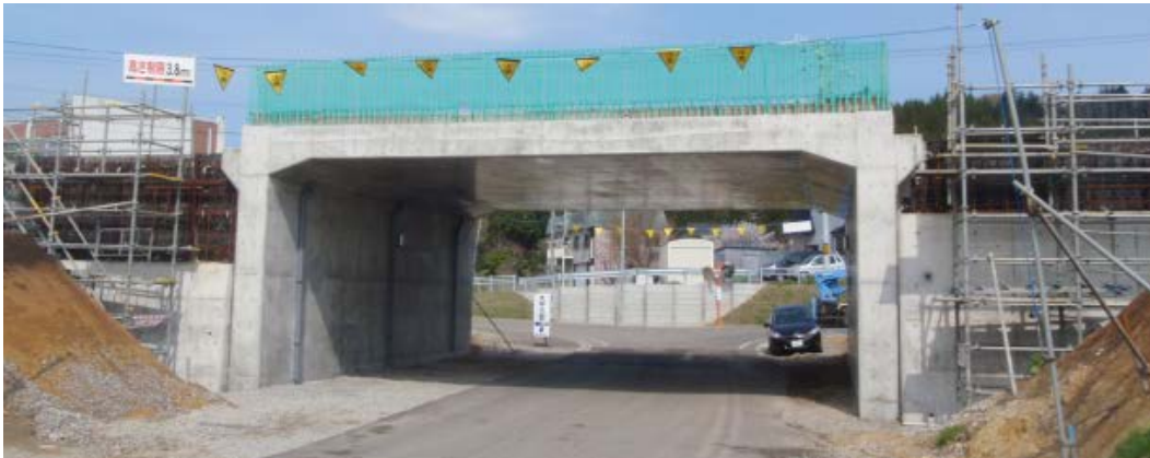
Fig. 13: First GRS integral bridge for a new high-speed train line at the south of Hokkaido: a) structural details (the width= 11.7 m); b) during construction (August 2011); and c) nearly completed (August 2012).
