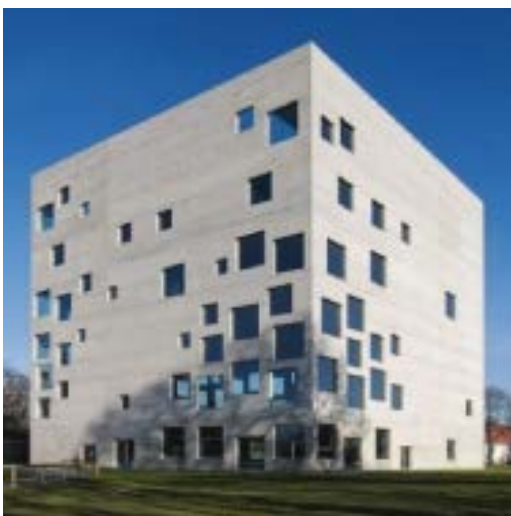
Fig.1: a) Zollverein School of Management and Design, Essen; SANAA, 2006: To keep the facade as thin as possible, the architects did away with conventional insulation in the building's outer walls. Instead, naturally available warm water is pumped through pipes set into the concrete, stabilizing the internal temperature ( http://www.domusweb.it/ ).
