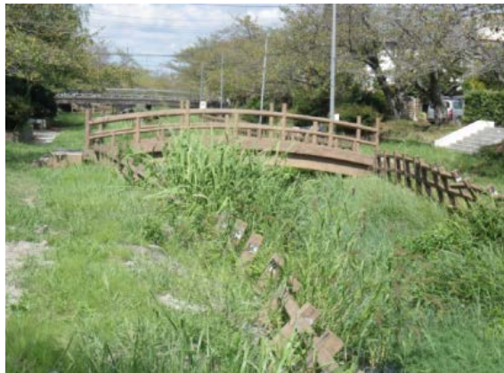
Fig. 6: Lateral flow of level ground facing at chanel in Katori city, Chiba prefecture
