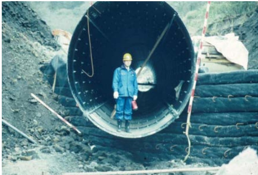
Fig. 3: Reconstruction works of railway embankment failure in Kyushu in 1991 by GRS RW technology [8]
