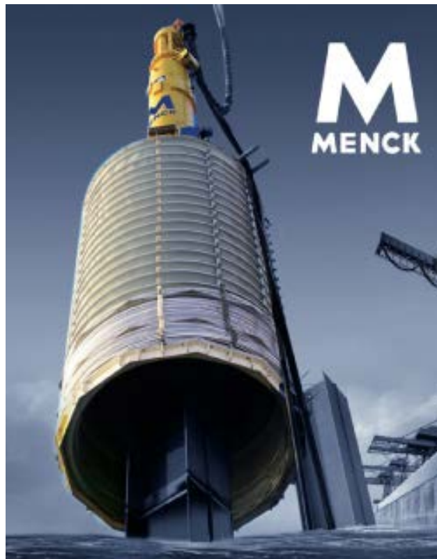
Fig. 16: Air bubble curtain around pile [13]
