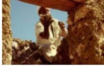
Fig (8.2): The walls are built using kershef natural material to keep the rooms cool
