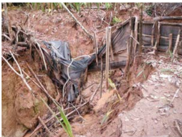
Fig.11 The outflow of the stored red clay
