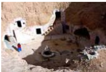
Fig. (4.1) Courtyards in Sidi Driss Tunisia, for climatic and defense
