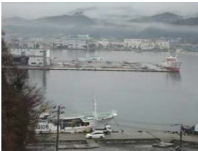
Fig. 1 Subsidence of lands, Kesenuma
