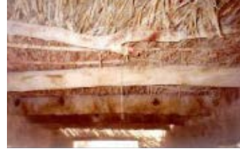
Fig (8.3): The roofs of the buildings are built from palm trunks which reduces heat gain inside the building
