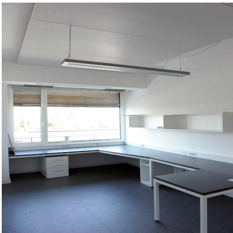
Illustration 3. The heating/cooling ceiling panels in refurbished offices.
