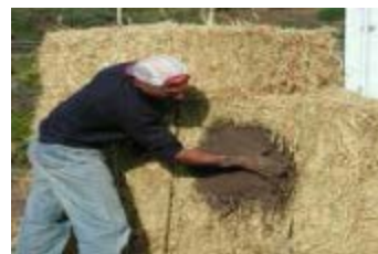
Fig (2.3): Building with straw bale
