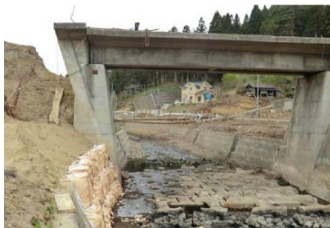
Fig. 7: Seaside view at Yonedagawa bridge in Noda village after tsunami affect, Iwate prefecture
