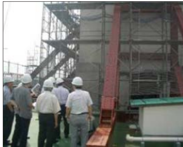
Repair of damaged building
