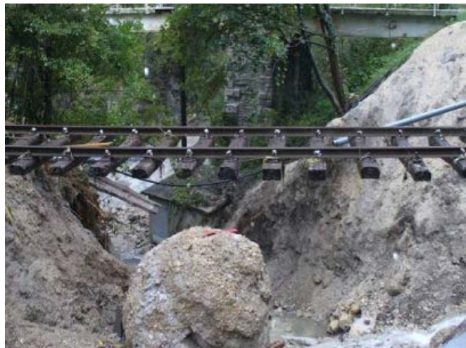
Fig. 2: Railway embankment that failed by rainfall and flood in September 2010 in Zagorje, Slovenia
