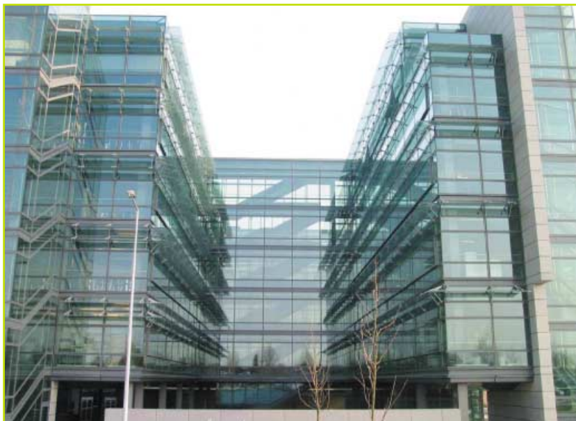
FIGURE 4 Chambre de Commerce with façade view and escape staircases in January 2004
