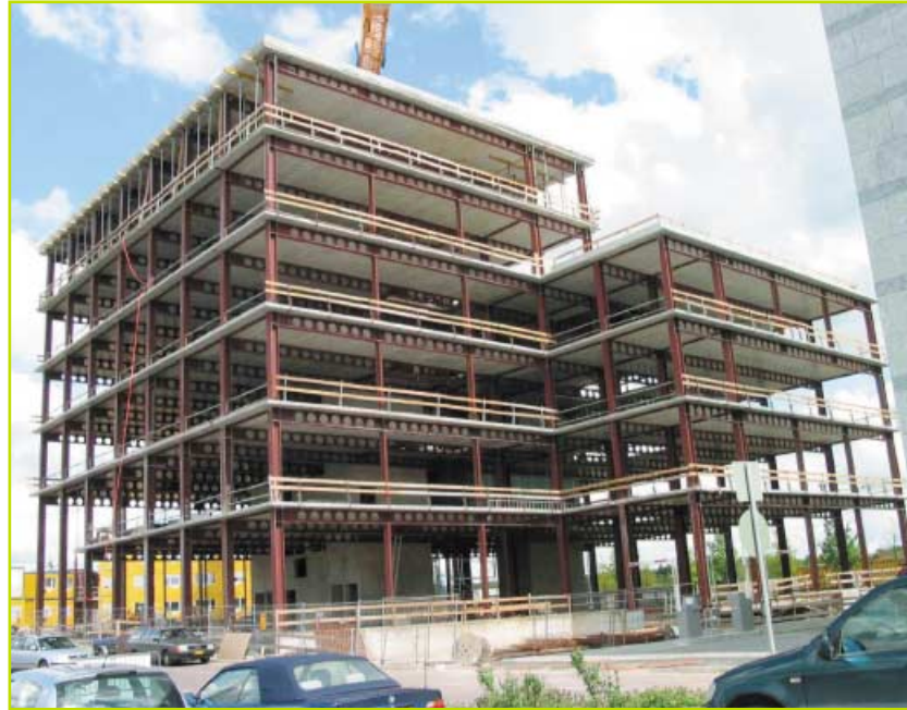
FIGURE 2 Banque Populaire with erected steel structure in May 2002
