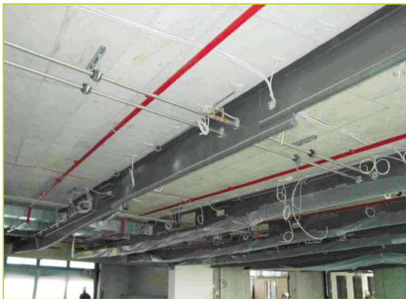
FIGURE 7 DEXIA-BIL building A, intermediate floor level with visible, unprotected composite beams
