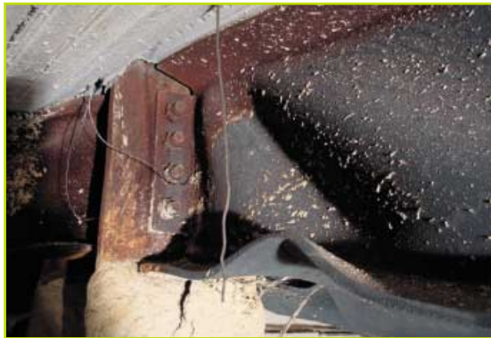
FIGURE 16: Beam web in shear
