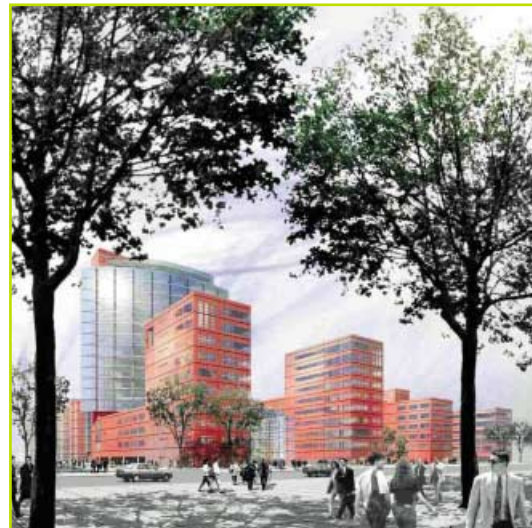
FIGURE 14 DEXIA-BIL buildings A, B and C as finished end 2006
