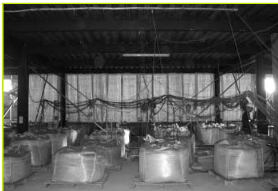
FIGURE 2: Sandbags on the 5 th floor
