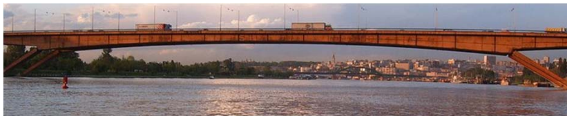
Gazela Bridge over Sava river
