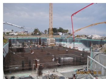
Figure 9 – Construction Stage 6 – Construction of raft foundation
