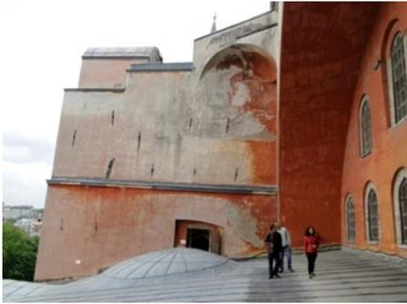
**Fig.7 Weathered red paint applied on the façades in 1986**
