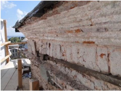
**Fig.3 Fossati ring at the base of the dome**
