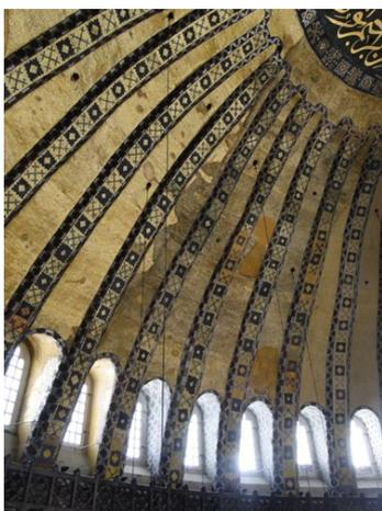
**Fig.4 The dome with deformed ribs**
