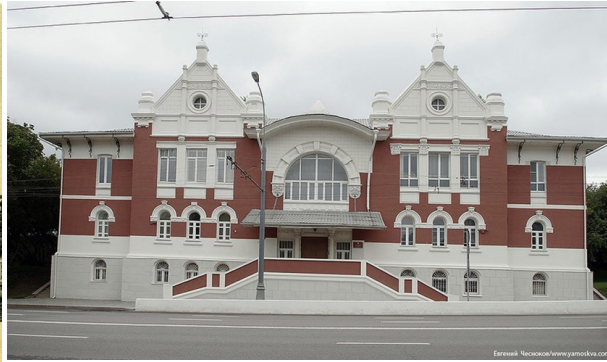
The building of the old terminal after the reconstruction in 2016
