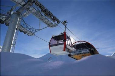
Kobi-Gudauri linking cableway covers over 7 km and is to serve 2800 passengers an hour. Considering that, the location of the route is on the northern slope enables skiers to enjoy skiing until the late spring. Implementation of one of the most complicated projects from engineering standpoint, took one year. Three cableways constructed with the 111 gondolas to connect with Gudauri cableway systems from Kobi by means of the stations.
