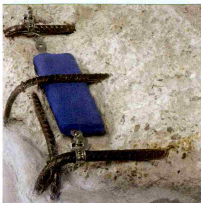
Vgradna anoda Mapeshield I
