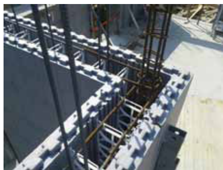
Slika 2 • Primeri vgradnje armature v ICF-stene evropskih ponudnikov, http://www.quadlock.com/concrete_forms/insulated_concrete_forms_construction.htm , 19. 12. 2016, https://laconstructiondesmarais.wordpress.com/tag/beton/ , 19. 12. 2016, http://maison-passive-alsace.blogspot.si/2012/07/coulage-beton-des-murs.html , 19. 12. 2016.
