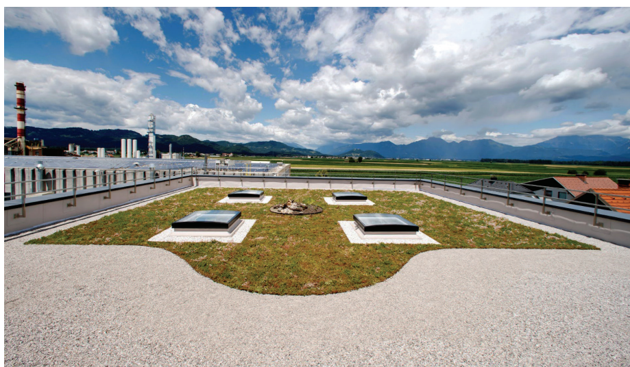
Slika 2 • Knauf Insulation Experience Center – zelena streha.
